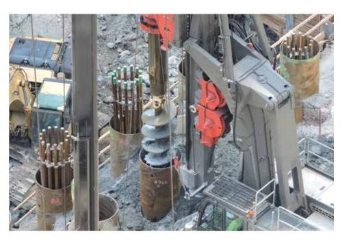
its on-staff engineering department, Skyline was able to design threaded bar caissons in 9-, 10-, and 13- bar varieties. These #28 threaded bar cages measured approximately 60 ft. in length, and fit inside both 36 in. and 48 in. OD x ½ in. wall pipe for the drilled shafts.
